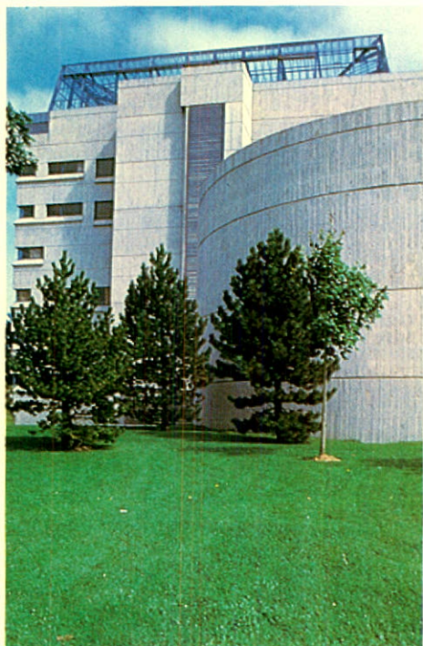
The Dalplex Sports Centre is part of the major construction project completed during 1982 at Dalhousie University in Nova Scotia. Canada Cement Lafarge was the sole supplier of the 2,500 tonnes of cement needed, and the building's inflatable roof structure was the first of its kind.
